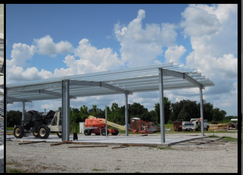
Tractor Shed under construction
